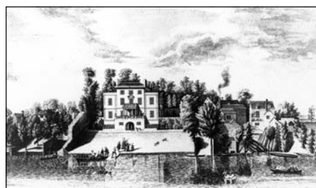
Pope's Villa and Grotto in 1735. The Villa has been demolished, but the Grotto survives behind a disused science laboratory
