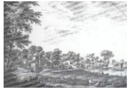
Muntz's view of the eclectic 'mabland' buildings of Radnor Gardens in 1756 showing the stream channel, since filled in 1970s
