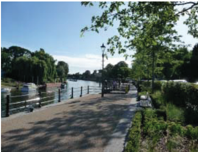
The southern embankment at Twickenham following restoration by London's Arcadia
