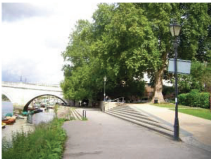
Restored steps at Bridge House Gardens
