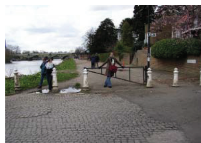
St Helena Terrace before restoration
