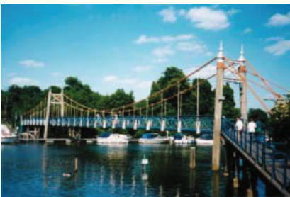
Teddington Lock footbridge
