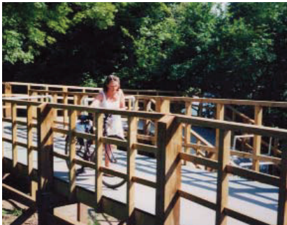
Accessible footbridge across Teddington Lock Island
