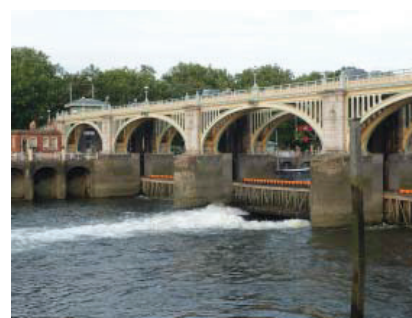
Richmond Lock and Weir
