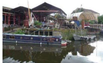
Boat repair facilities at Brentford
