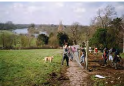
Volunteers removing the unsightly chain link fence on Richmond Hill
