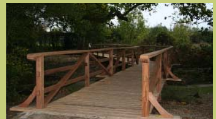
Douglas Meadow: Boardwalk after construction
