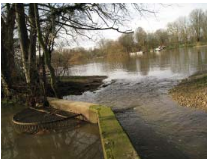
Some stretches of the riverbank are continually eroded by the tides
