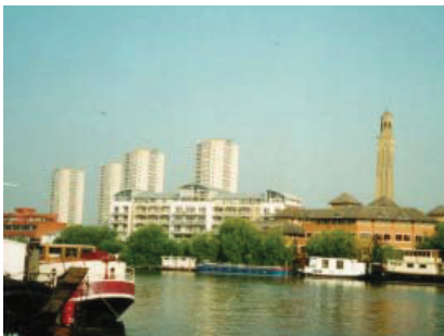
The tower of the Steam Museum soaring over new developments at Brentford
