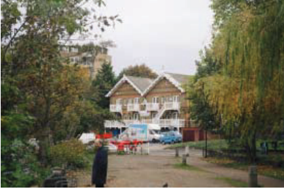
The converted boathouses at Lower Ham Road, Kingston
