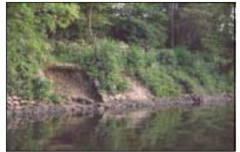
Banks are subject to erosion from boat wash
